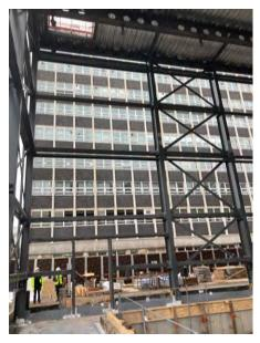
The steel frame of the central core and chambers are nearing completion, and the chamber floors are starting to take shape with gas membrane nearly complete and ready for topping with concrete.
